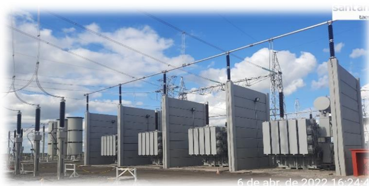
Transformers for the Synchronous Compensator SE Livramento 3 – Sant'Ana
